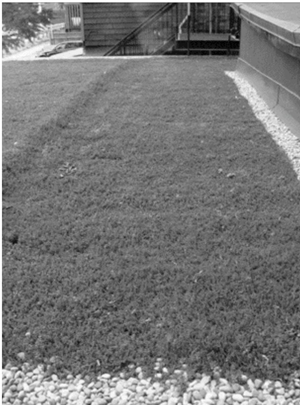
Figure One: The rooftop of the Gladstone Hotel
